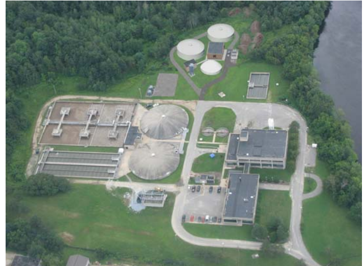
This engineered aerial view shows the existing LAWPCA WWTP in the lower 2/3rds and the to-be-built digester complex at the top.
